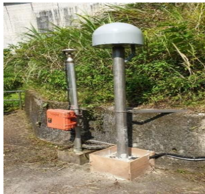
GNSS monitoring station in the left abutment
