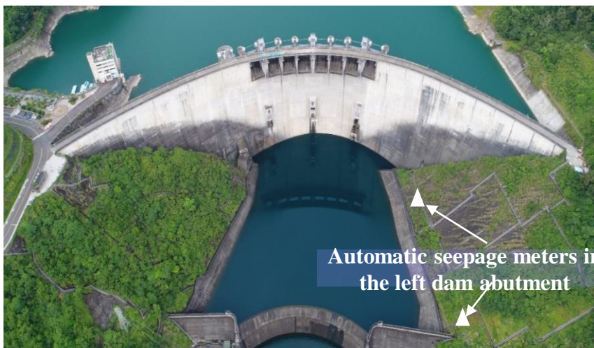
Location of the automatic seepage meters in the left abutment
