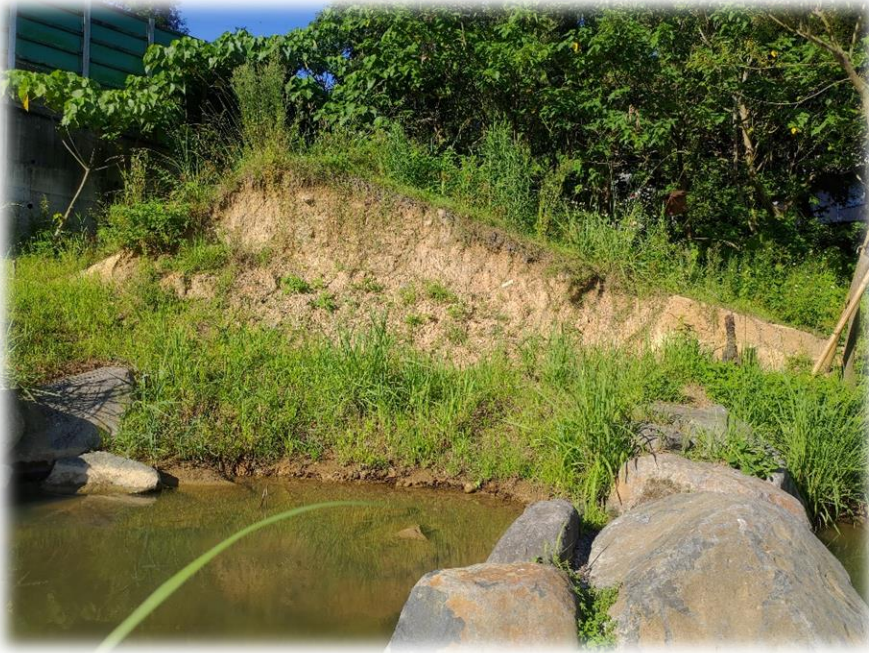
kingfisher earth embankment
