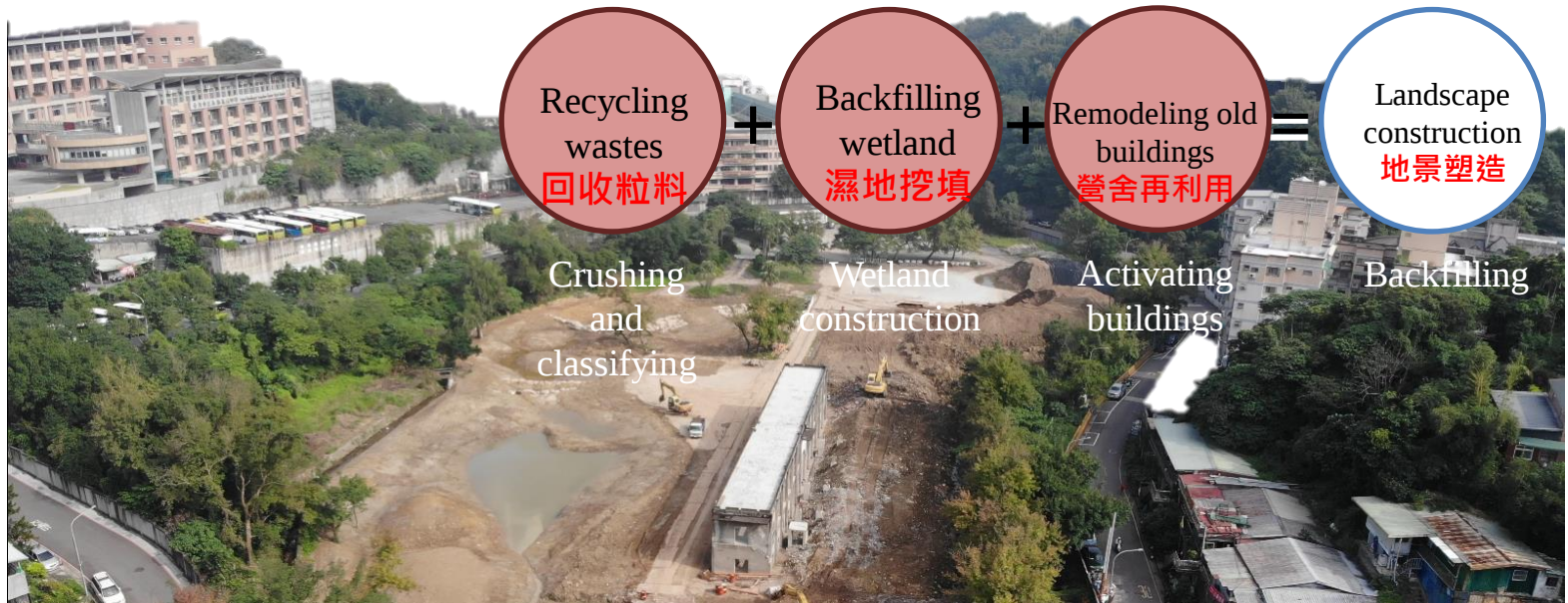
Classifying and crushing backfilling materials
