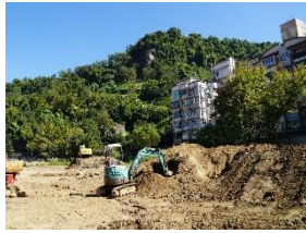
Backfilling with on-site soil
