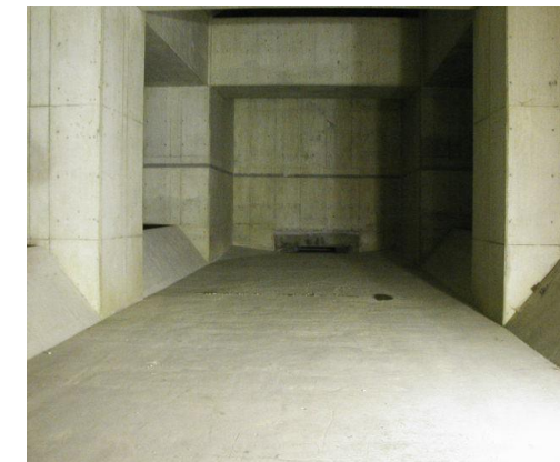
▲ Minamisuna Rainwater Reservoir with multiple dwelling units above for the effective use of space (storage capacity of 25,000 m 3 )
