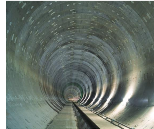
▲ Wada Yayoi Trunk Sewer provided along the Kanda River, which floods extensively (inner diameter of 8.5 m; storage capacity of 150,000 m 3 )
