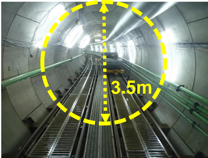
Sewer for storing rainwater (Tagara and Sakuragawa, Nerima Ward)
