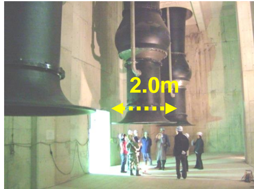
Pumps for rainwater (Kamiya, Kita Ward)
