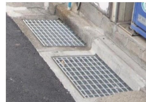
Additional catch basins
