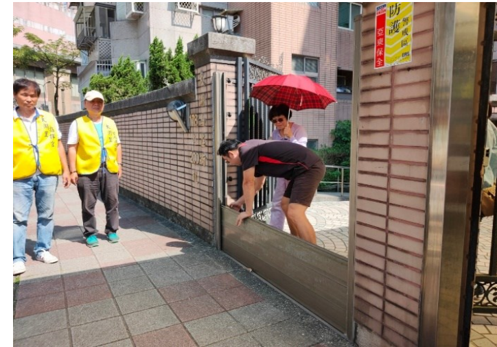
Erecting flood gates
